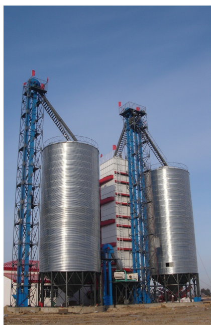
Figure 11. Rice Downflow/Counterflow Drying Equipment with a Capacity of 500t/d
