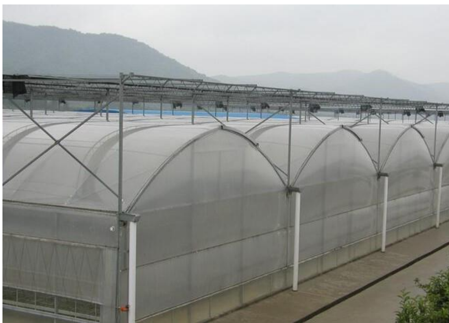
Figure 2-2 Appearance of the continuous greenhouse
