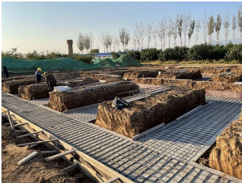
Figure 1-38 The foundation of a chicken house
