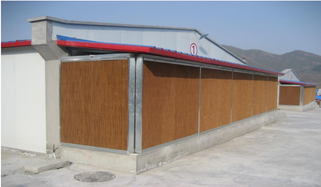
Figure 2-8 Wet pad cooling house Yukou
