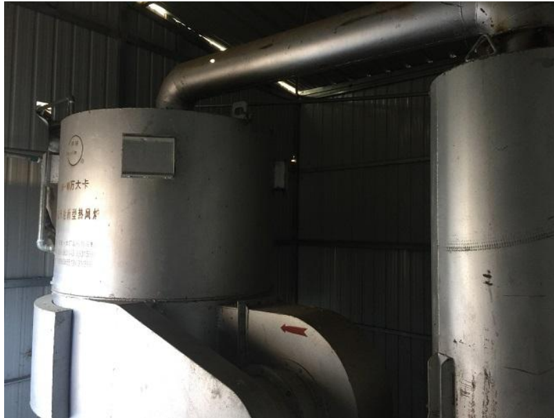
Figure 2-1 Hot-Air heater
