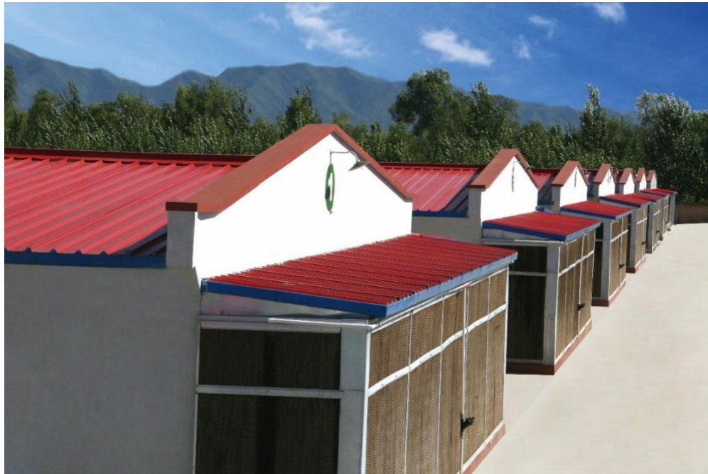
Figure 2-8 Wet pad cooling house Yukou
