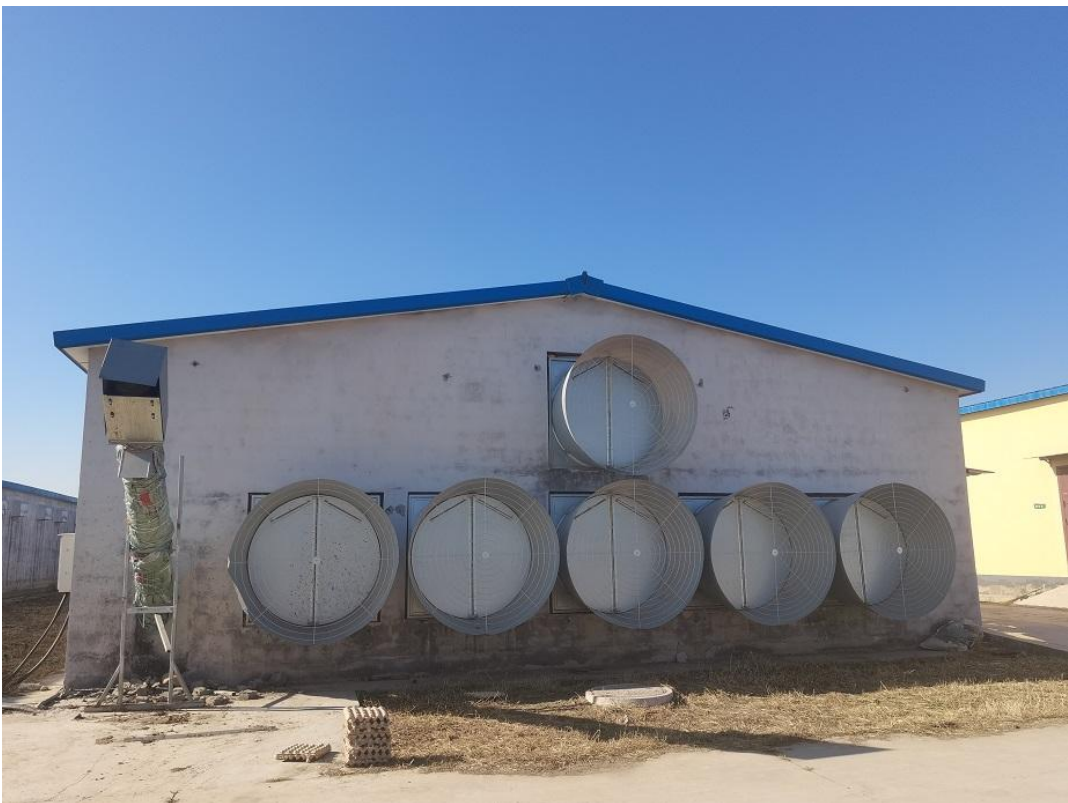
Figure 2-13 Longitudinal ventilation, Zunhua
