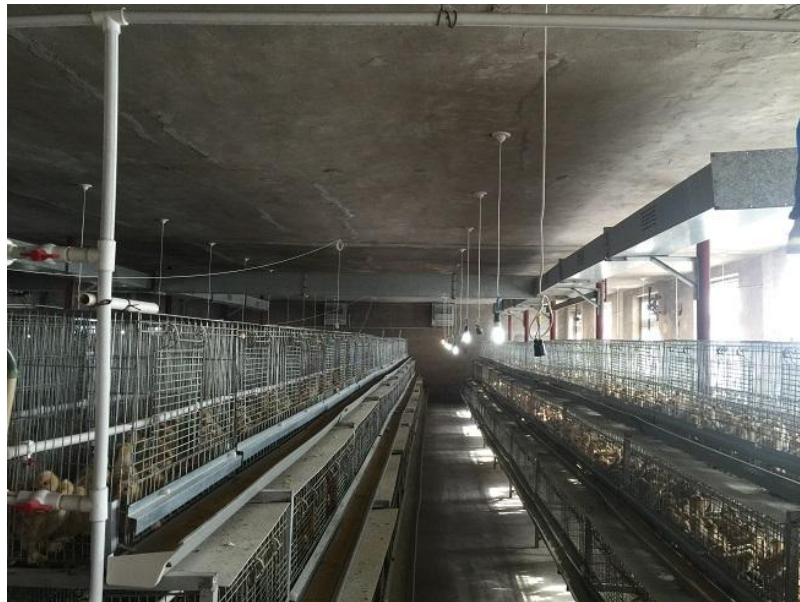
Figure 2-2 Hot air heater house
