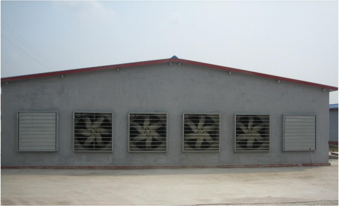
Figure 2-12 Wet pad cooling house Yukou
