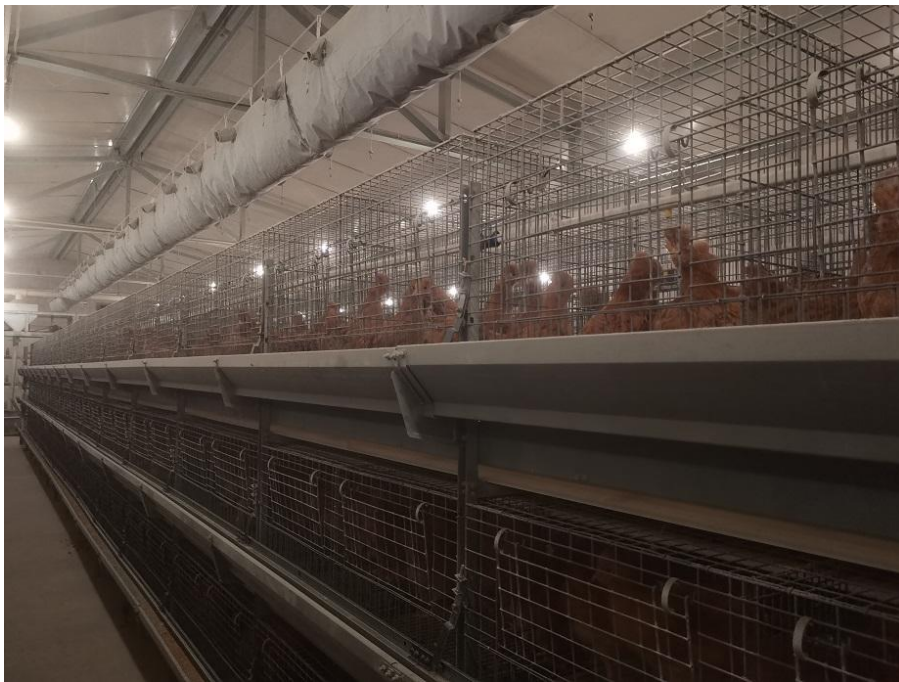
Figure 2-31 The brooding cage using the hot air system
