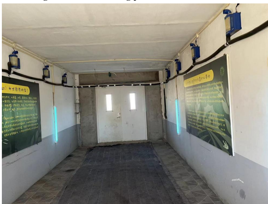
Figure 1-7 Disinfecting room between the living area and production area
