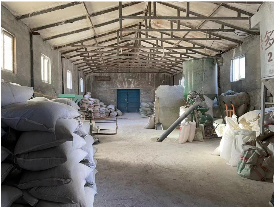
Figure 2- 54The feed plant in chicken farm
