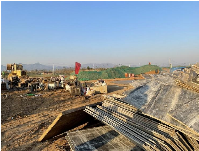
Figure 1-40 The construction site of a chicken house
