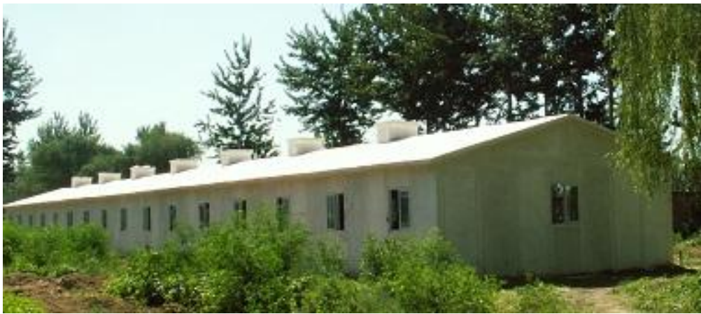
Figure 1-38 The chicken house with natural ventilation
