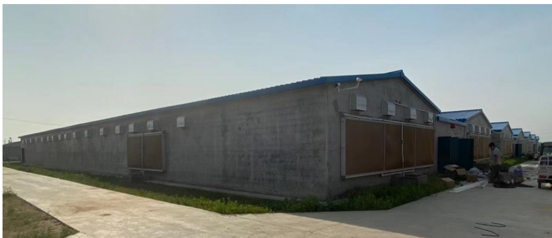
Figure 1-37 The chicken house with wet curtains and fan system
